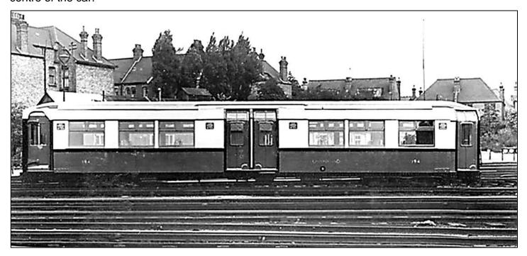
Figure 2: Hampstead gate stock trailer car No. 194 in the yard at Ealing Common depot after its conversion to air door operation. The two end platforms have been enclosed and side doors provided while a double doorway has been cut in the centre of the car. The layout was similar to the 1920 Cammell Laird stock. The door on the west end of the car is a special design to test the concept of a rotating door rather than a sliding door. Photo: LT Museum.
