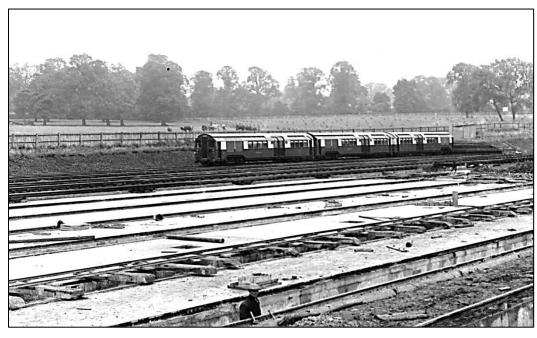
Figure 1: Morden depot about mid-1925, showing three 1924 Met. Carriage motor cars stored on No.1 road after delivery. depot is a long way from complete. They have dug the pits and concreted some of them but they haven't put up any of the building structure Storing cars for long periods leads to quite rapid deterioration and I suspect some cars needed work before they were fit for service. Photo: B.R. Hardy collection.
